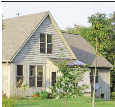
Richard Stumpner's home in Bloomington has a passive solar system. Eventually the trees will shade the south side of the house in summer but allow the sun in during winter. Photo courtesy Richard Stumpner
