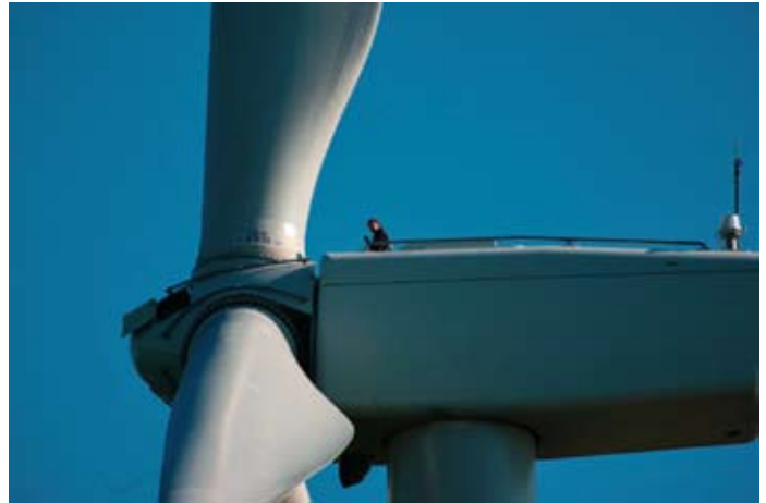
Work being done on a wind turbine at the Benton County Wind Farm (Photo by Tom Campbell, Purdue University)
